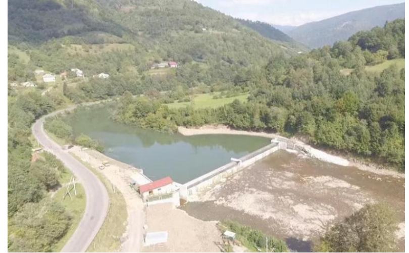
Water intake structure with “fish ladder” of the Nizhniy Bystryi SHPP-2 (232 kW) (photo by O. Stankevich-Volosyanchuk)
