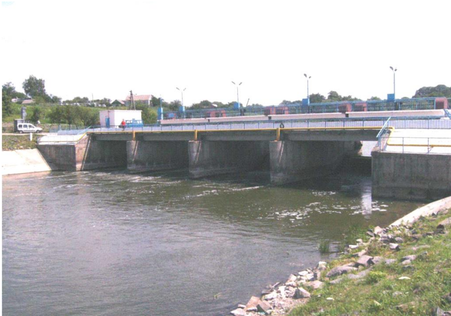
The sluice-regulator near the village of Voskodavy
