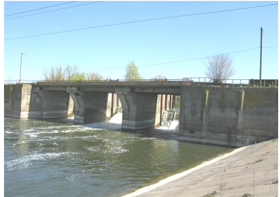
The sluice-regulator near the village of Metkiv
